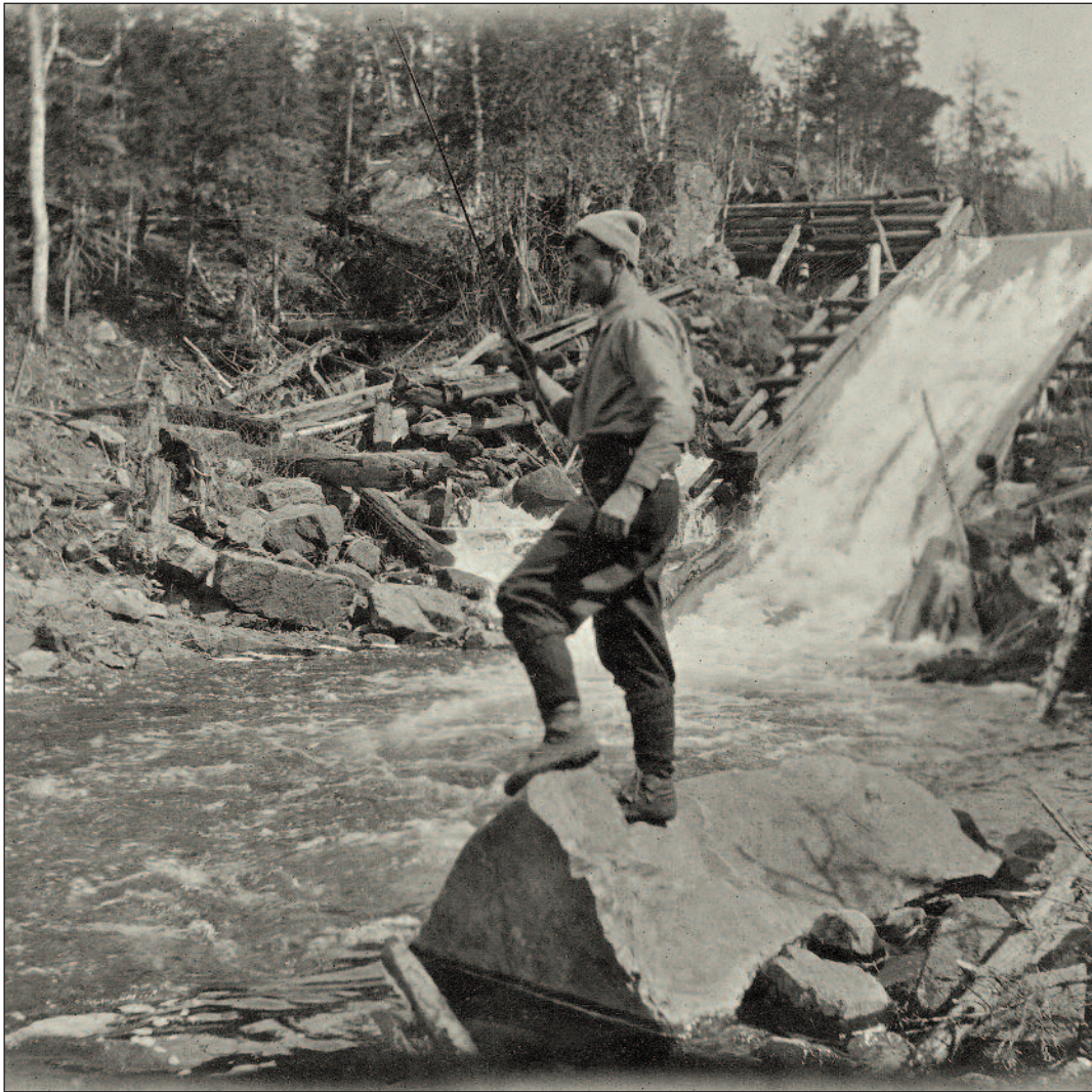
This photo of Tom Thomson at Tea Lake Dam verifies he was a fly fisherman, at least some of the time, when circumstances suited. He is clearly using a fly rod and is apparently stripping in line. Unknown photographer, Tom Thomson at Tea Lake Dam, ca. 1916, 10 x 10 cm (3 15/16 x 3 15/16 in), Art Gallery of Ontario, gift of Marjorie Lismer Bridges, 1976, LA.ALF.S5.1. With permission.
