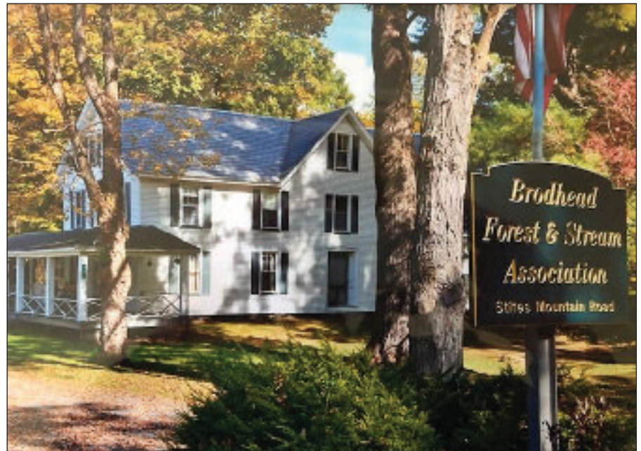
Built in 1860 to accommodate more guests at the Stites Mountain House, the annex now contains an equipment room, a fly-tying room, and various sleeping rooms for club members and guests.
