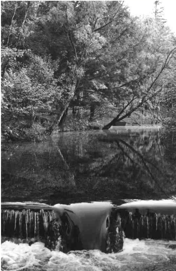
The spillway at Stapler Dam, the home pool.
