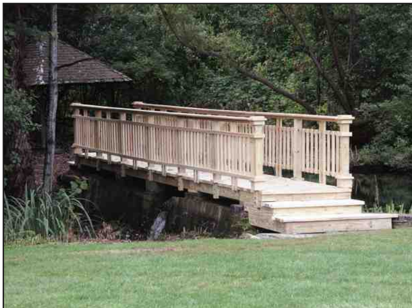
The museum's newly repaired bridge.
