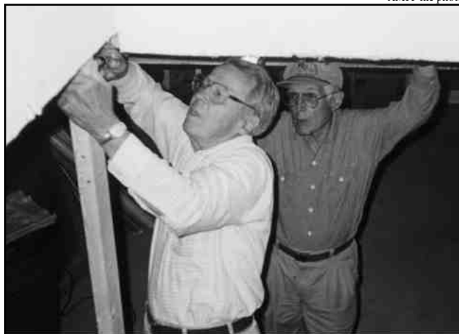
Ted Ferree (left) and Dick Finlay work in the basement of the museum's Seminary Avenue home.
