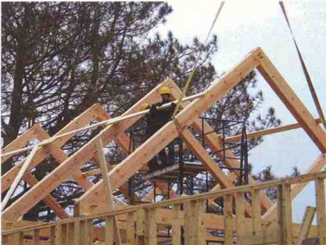
Undeterred by February's cold temperatures, workers pieced the framework together.
