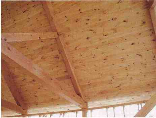
A close-up view of the gallery ceiling from inside.
