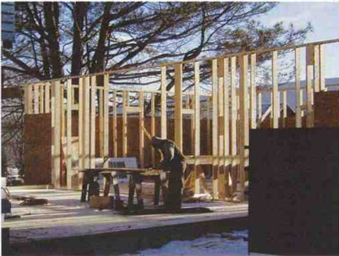
The gallery walls started going up in late January.
