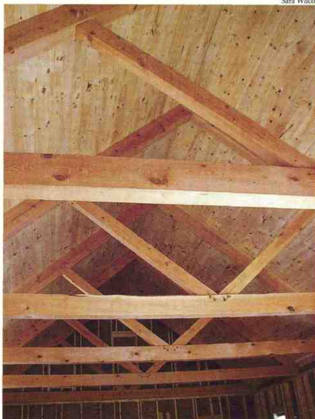
Timber-frame ceiling of the Museum's new gallery space.
