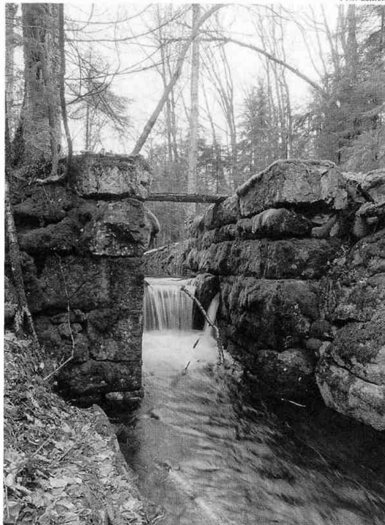
Dam at Canachagala Lake, constructed by New York State in 1881 to impound water for the Black River Canal, shown in 1989.
